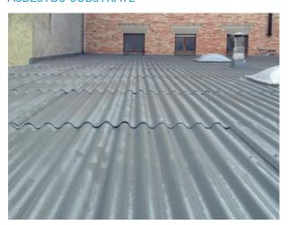
In many cases the overlaps of the plates that make up the substrate need to be resealed using TECNOFOAM sprayed polyurethane rigid foam (depending on the amount to be applied), as well as checking their overall condition. Likewise, any screws, nuts and bolts in bad condition need to be resealed using MASTIC PU polyurethane Mastic or TECNOBAND 100 (see technical specifications on TDS).
