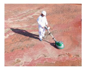
You will need also the grouting the joints or sores of the ceramic pieces, and cleaned and repair the existing expansion joints by removing the existing material, cleaning, filling with MASTIC PU, and band placement TECNOBAND 100 (see technical specifications for these products) at the top.
